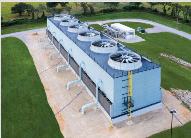
Vista Ridge Water Transmission Project, San Antonio
